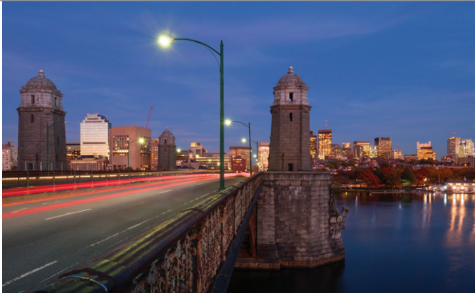
Longfellow bridge from Cambridge to Boston at night (photo: The StressCrete Group)
