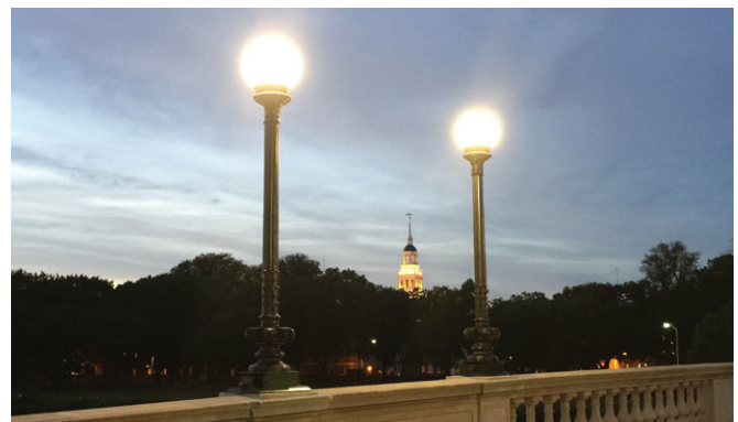
John Weeks bridge from Cambridge to Boston at night (photo: The StressCrete Group)
